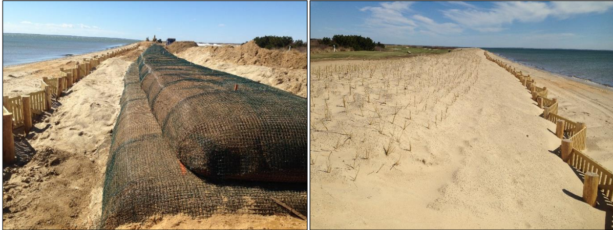
Figure 82. Example of a coir project on Cape Cod, located in NHESP habitat.
