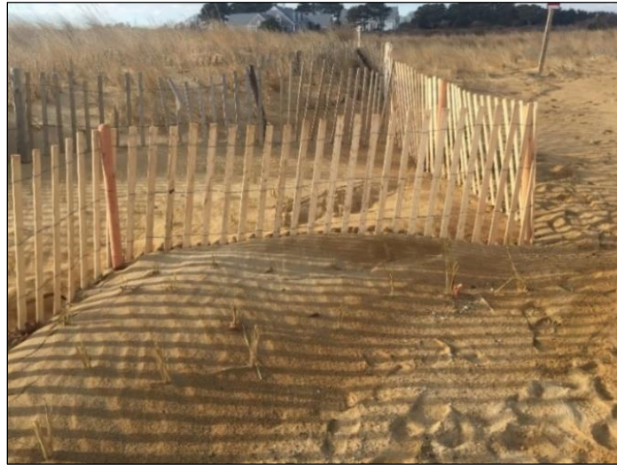
Figure 84. Example of wind-blown accumulation at the base of drift fence in Edgartown.
