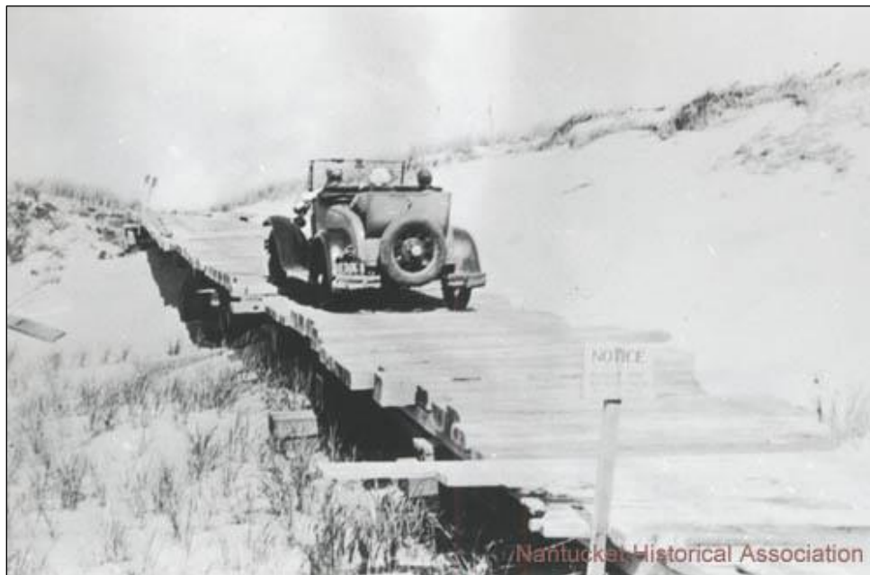
Figure 62. Photograph of Model A driving over timber roadway into the dunes (Image courtesy of the Nantucket Historical Association).
