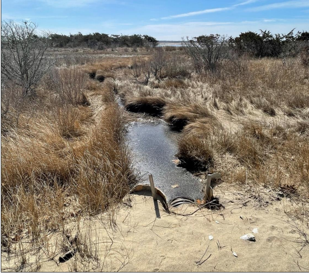
Figure 45. Existing corrugated plastic pipe under road.
